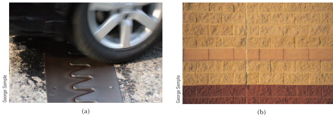
Figure 19.7 (a) Thermal-expansion joints are used to separate sections of roadways on bridges. Without these joints, the surfaces would buckle due to thermal expansion on very hot days or crack due to contraction on very cold days. (b) The long, vertical joint is filled with a soft material that allows the wall to expand and contract as the temperature of the bricks changes.
